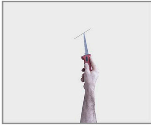
Step 2- Cut out opening in Drywall. *Review Project submittal for exact cutout dimension requirements.
