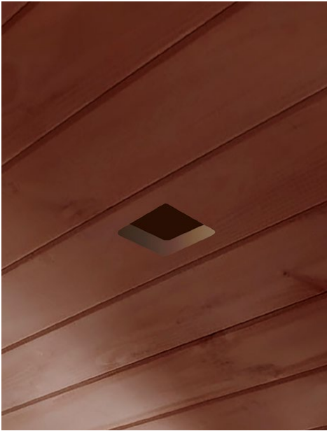
Step 1- Cut opening to fit housing installation. (see drawing below for specific cutout size details).
